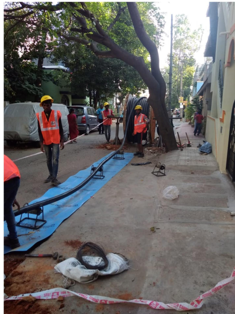
Pic 12: Underground cabling work
