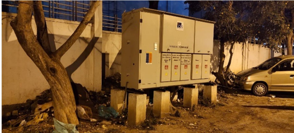
Pic 1: Installed RMU
