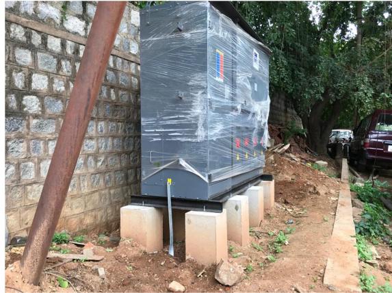
Pic 10: Installed RMU
