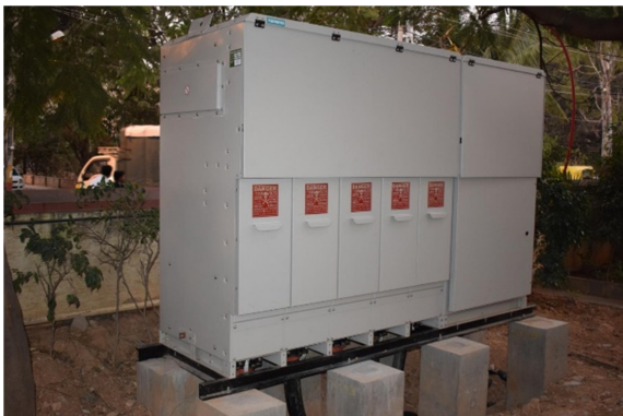
Pic 7: Installed RMU
