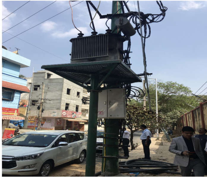
Figure 21: Pole Mounted Transformer
