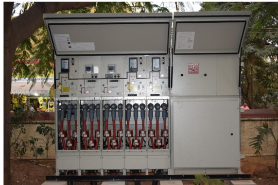
Pic 6: Installed RMU
