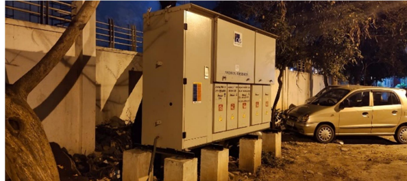
Pic 2: Installed RMU
