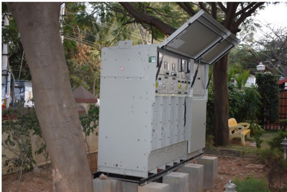
Pic 5: Installed RMU
