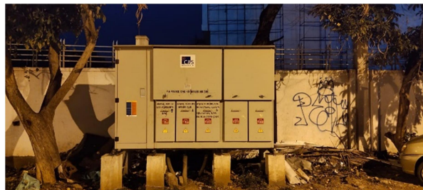
Pic 4: Installed RMU
