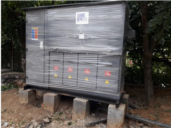
Pic 9: Installed RMU
