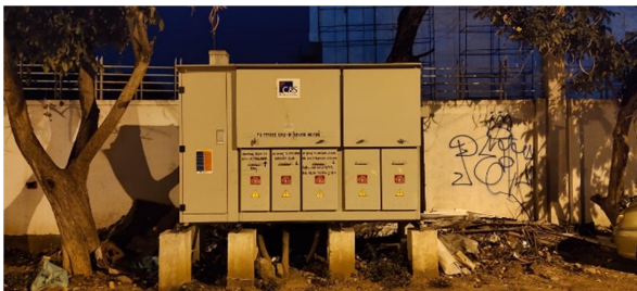
Pic 3: Installed RMU
